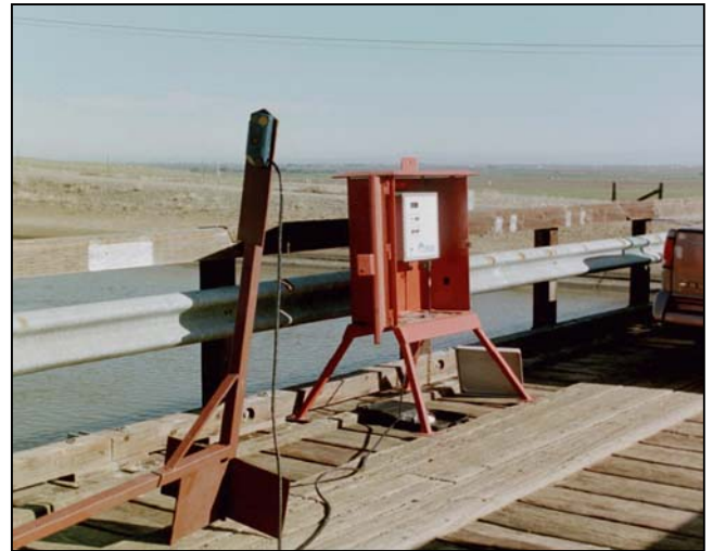
Figure 3. Doppler Unit at Head of Delta Mendota Canal Prior to Installation
