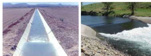
Figure 1. Replogle flumes in irrigation canals
