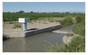
Figure 3. Rectangular Replogle flume with tapered entrance and smooth rounded edges (Truckee-Carson Irrigation District)
