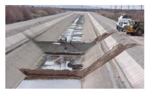
Figure 2. Trapezoidal Replogle flume in existing concrete lined canal
