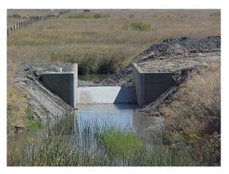
Figure 5. Constructed rectangular Replogle flume
