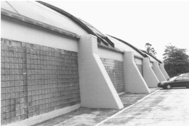
Fig. 8. Exterior view showing edge beam (photo by David Billington)
