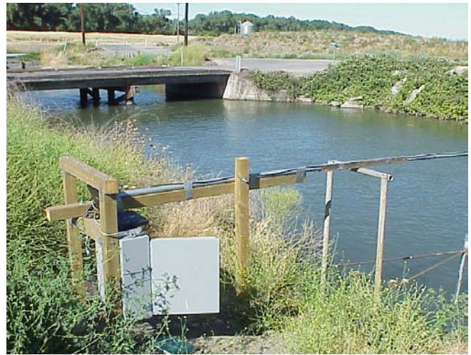
Figure 3. Tisdale Main Canal
