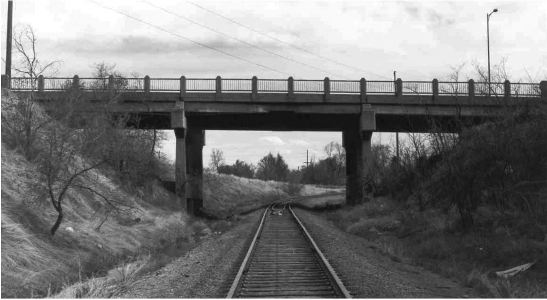
Fig. 1. Colorado State highway bridge E-17-AH
