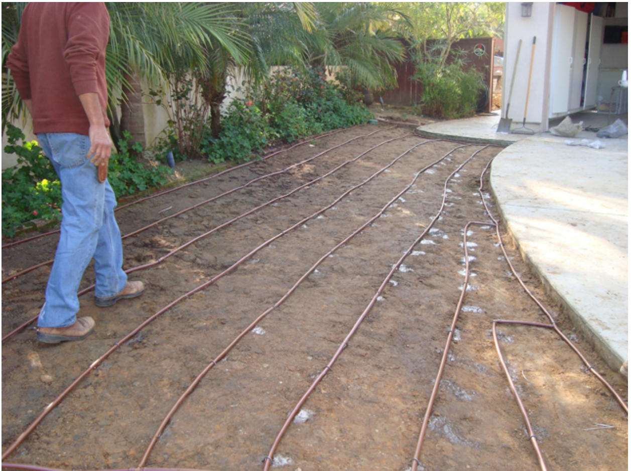
FIGURE 11. Subsoil Irrigation System Installation. Source: Advanced Greywater Recycle Systems (2012).
