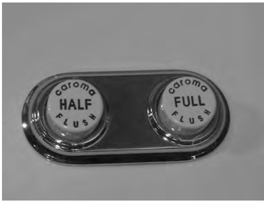
Figure 1 – Dual Flush Toilet
