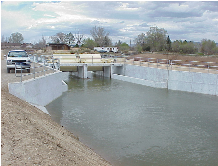
Figure 4. Typical Installation of Automatic Radial Gates and Long Crested Weirs
