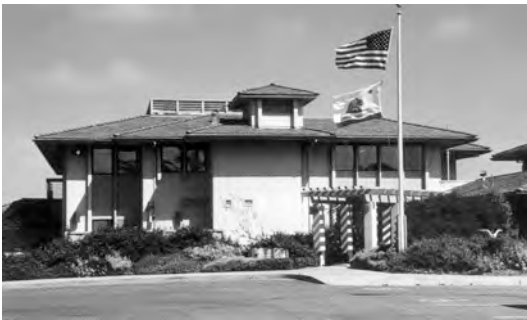
Figure 4 – Education Building at the Monterey County Regional Waste Management District
