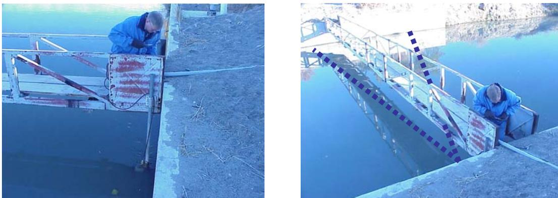
**Figure 4. SonTek/YSI Argonaut SL installed in a canal**
