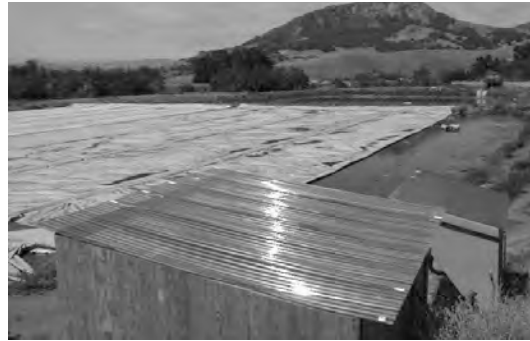
Figure 4 – Cal Poly Covered Dairy Lagoon Digester After Williams, D.W. and D. Gould-Wells, 2003
