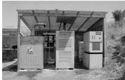
**Figure 5 – Cal Poly 30kW Microturbine Installation**
