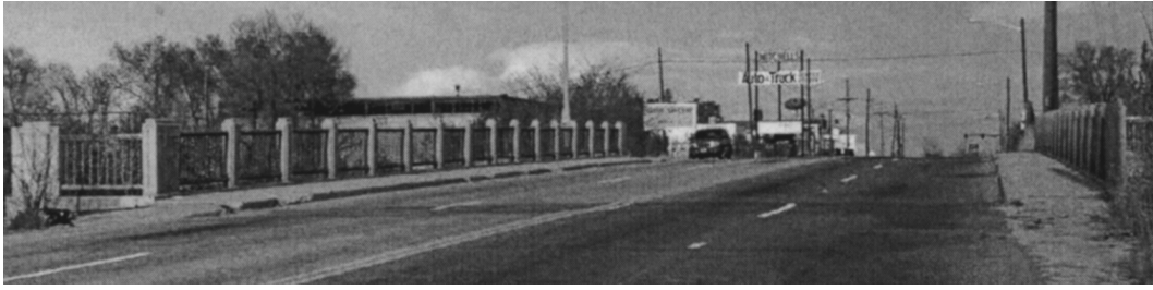
FIG. 2. Bridge E-17-AH-Roadway and Railings
