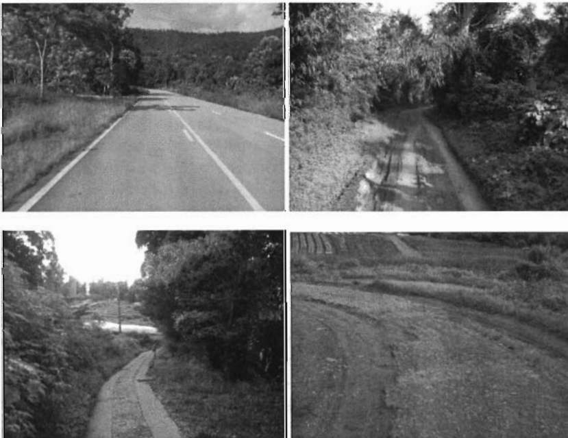
Figure 4. Various road conditions measured in this study.
