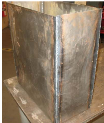
Figure 14: Reservoir with 5 walls welded
